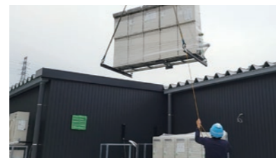
A pre-assembled water heating system delivered to a construction site
