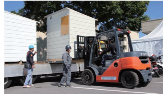
Installing a shower booth at an evacuation center
